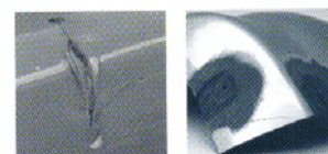
Repairing damaged plastic
