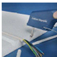
Cutting U-channels for embedding cables
